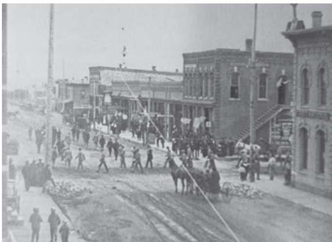
Intersection of 5th and Main Street, looking east. Mid-1890s
