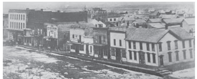
4th and Main Street view looking southwest. The Merchant's Hotel is located on the far left. All buildings facing the street burned down in 1888.
